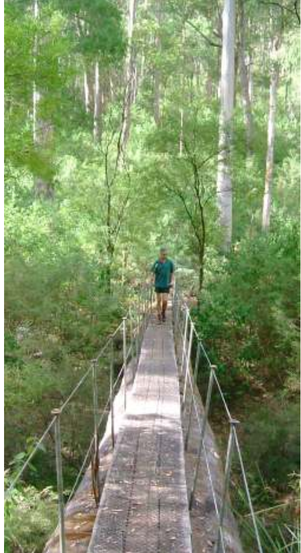
The bridge over the Donnelly River
